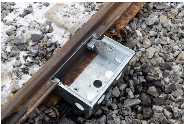
Installed box at separated groove, still without an axle counter.
