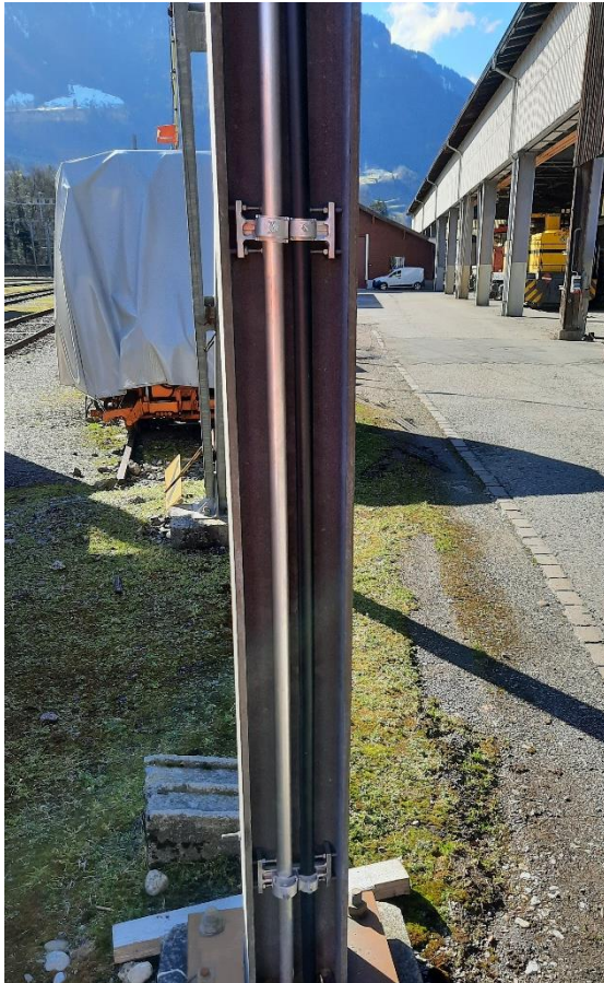
Fast fastenings visible in the pictures: 32-40mm (on the left) and 25-32mm (on the right)
