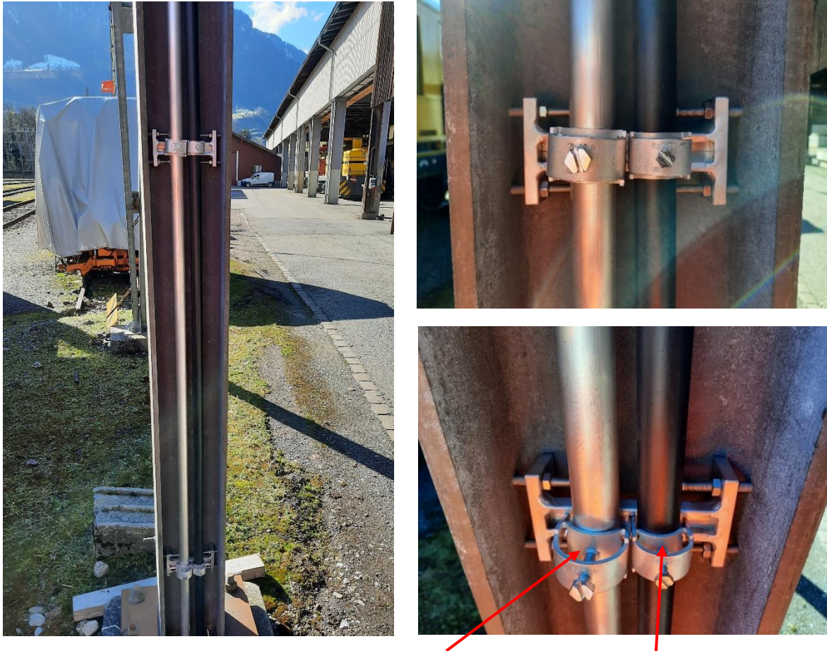
Fast fastenings visible in the pictures: 32-40mm (on the left) and 25-32mm (on the right)
